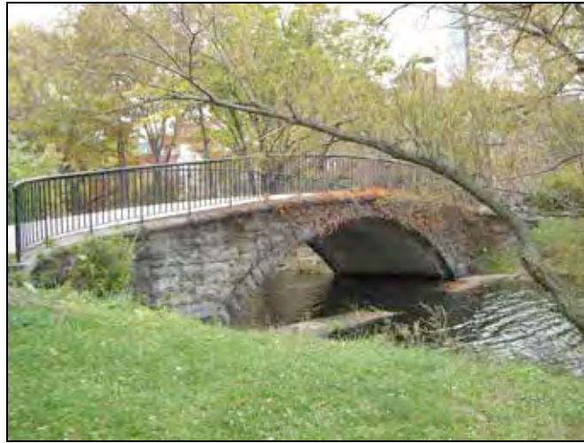
Figure 6.35 – Original granite bridge with new railing.
