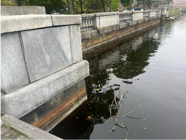
Commissioners Landing balustrade.
