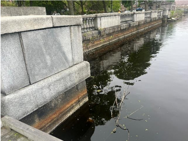
Commissioners Landing balustrade.
